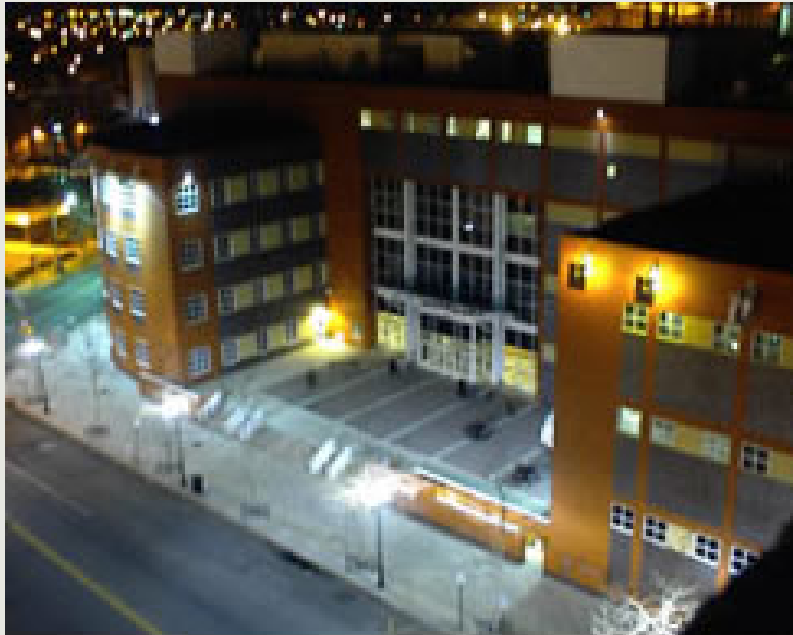
Exterior of Civic Square Building
