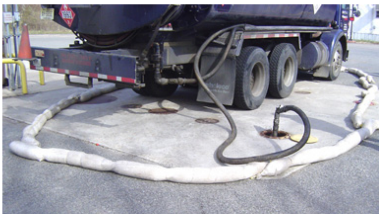
Spill Prevention Control and Countermeasures deployed during fuel delivery on Busch Campus.
