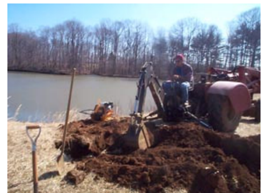
Repairing dam at Cream Ridge Farm
