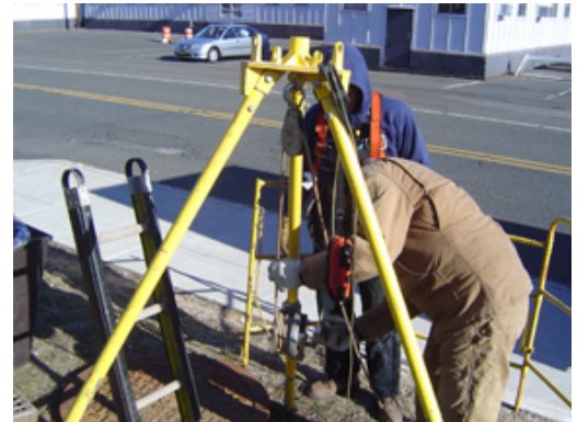
Utilities personnel preparing to enter into a confined space.
