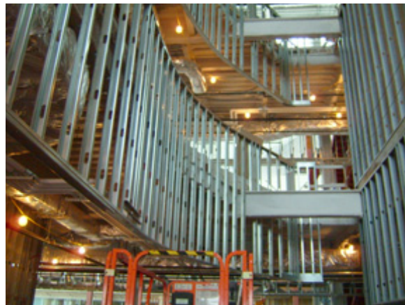
Construction of Biomedical Engineering Building on Busch Campus.
