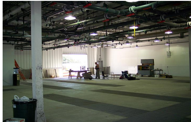
Southeast corner of hatchery building
