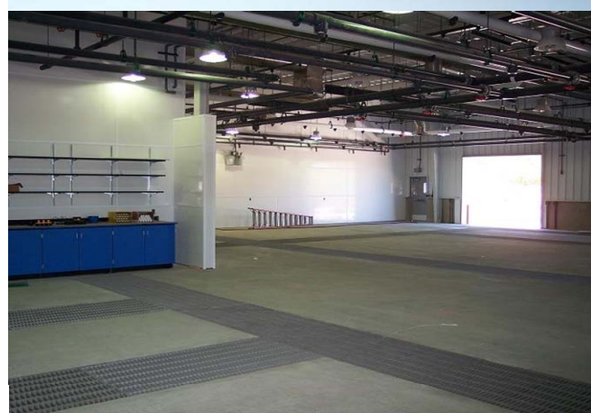
Southwest corner of hatchery building
