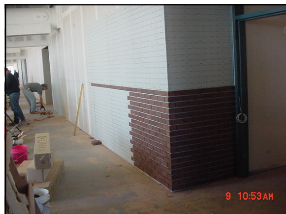
Thin Brick Corridor Walls
